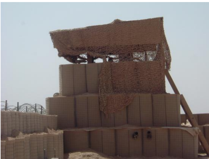
Royal Engineers complete the camp security tasking
